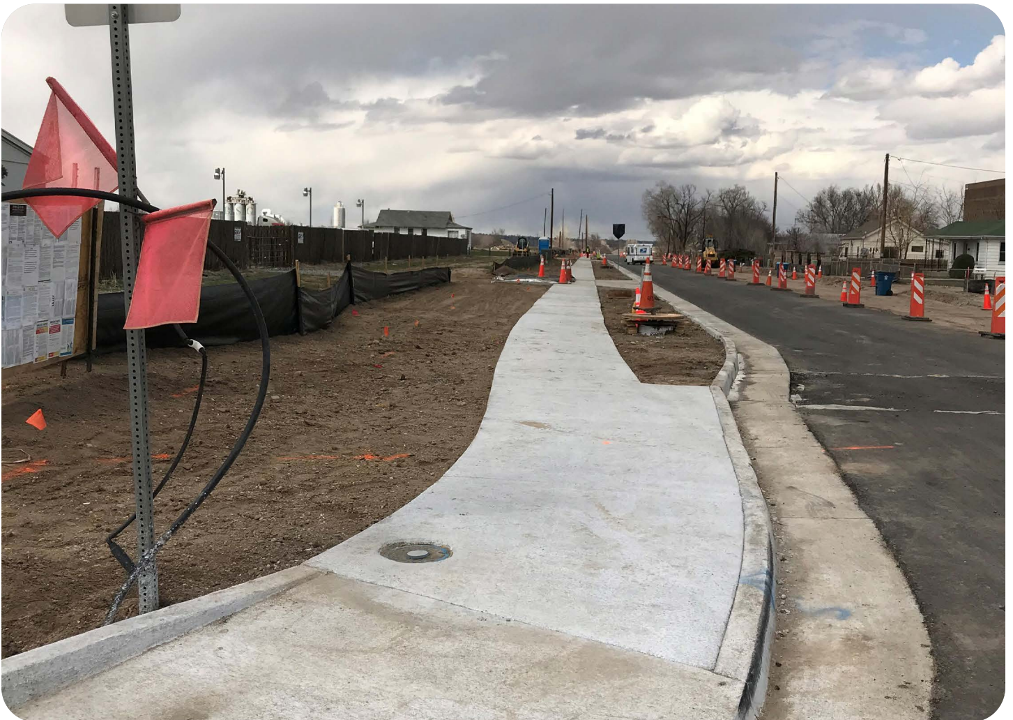
When streets and roadways are widened and reconstructed, sidewalks and curb ramps must be brought into compliance with Americans with Disabilities Act standards. Photo credit: Commerce City
