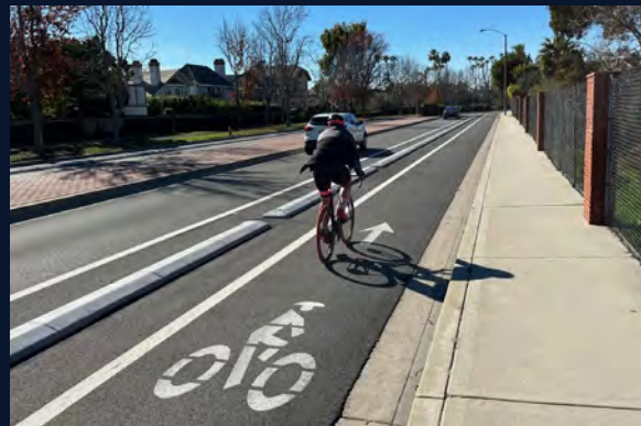
Protected Bike Lane
