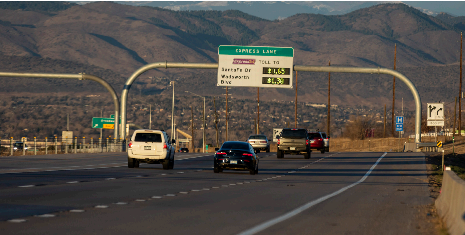
C-470 at University Boulevard in Highlands Ranch. Photo by Stephen Martinez/Colorado Department of Transportation
